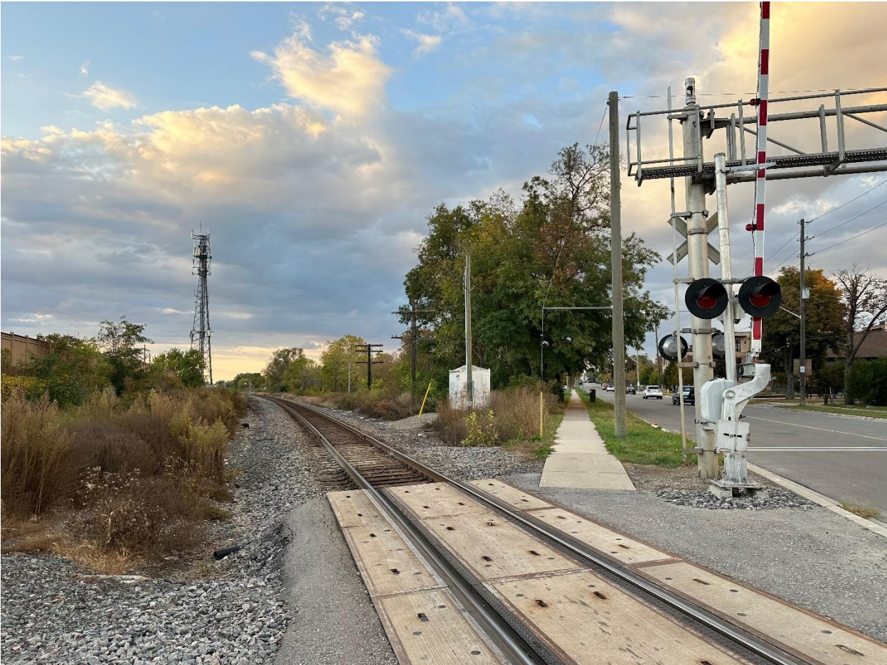
Figure 7: Kipling Avenue at the CPKC MacTier Subdivision crossing looking north
