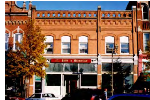
Historic commercial design, this example from Collingwood: The shopfront forms the base, the wall forms the body, and a wide fascia and cornice forms the cap.
