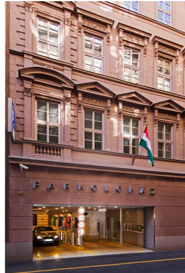
Figure 34– Parking structure as part of urban fabric
