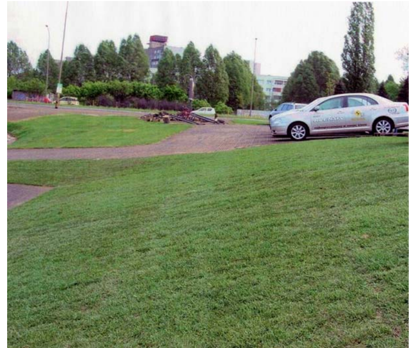
Figure 24 – “Green” parking lot supported by root cell structure
