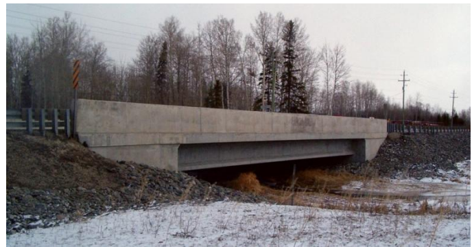
Figure 6. Example of a Concrete Box Girder Bridge
