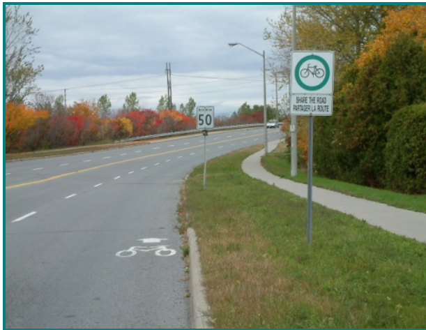
Example of Signed-Only Bicycle Route with a Wide Curb Lane and bicycle route pavement marking – City of Ottawa
